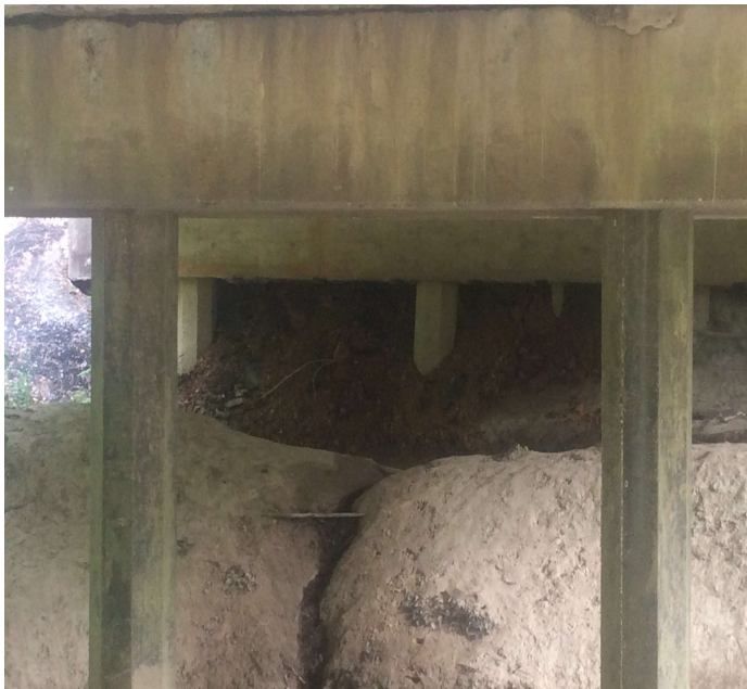
PHOTO 1 Description Scour under abutment 2
