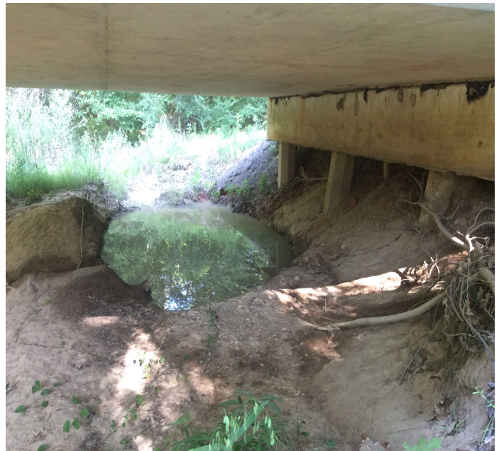
PHOTO 2 Description 05364 scour hole under span 3 columns 1-3 shown .
