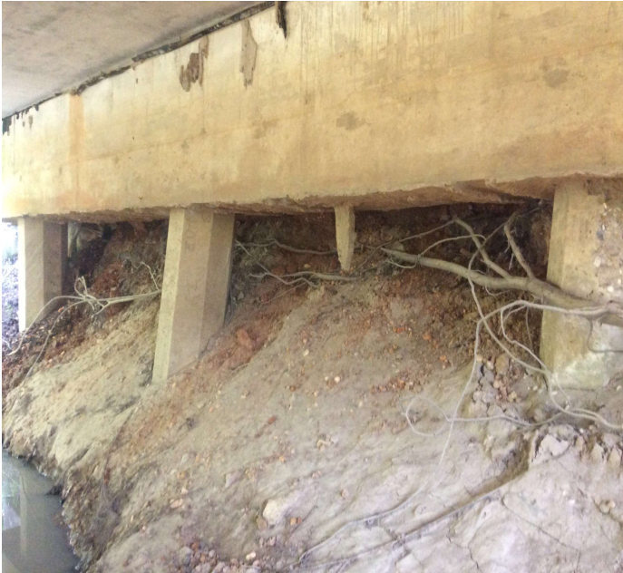
PHOTO 3 Description Abutment 2 erosion
