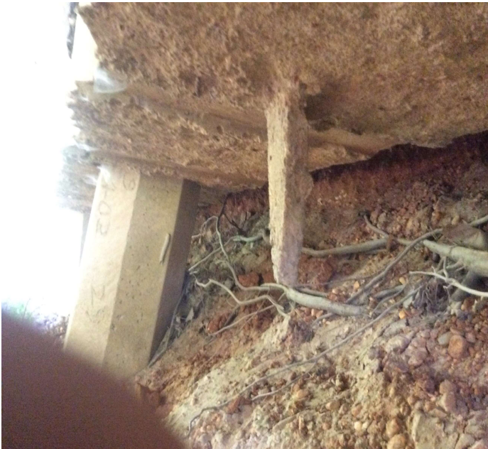
PHOTO 4 Description Erosion abutment 2
