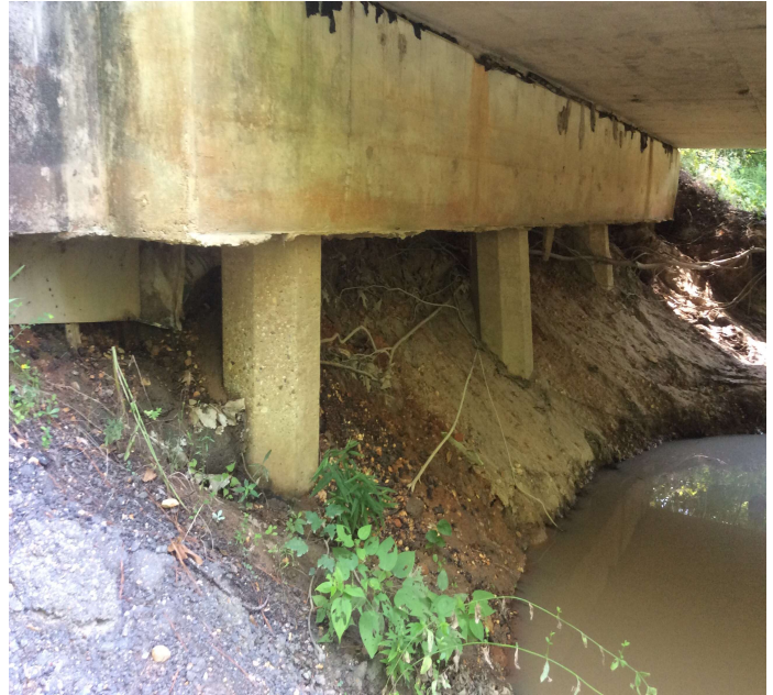
PHOTO 5 Description Abutment and slope erosion note visible aggregates column 1
